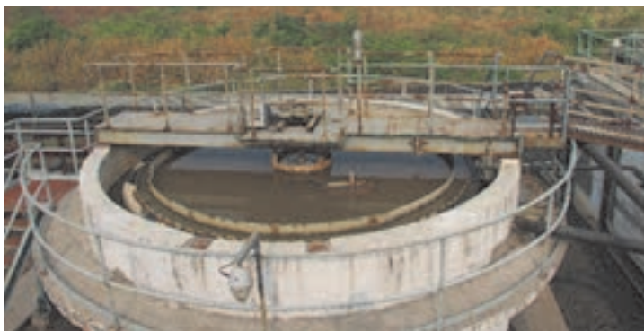
Our waste water treatment plant at GIL Ambernath
