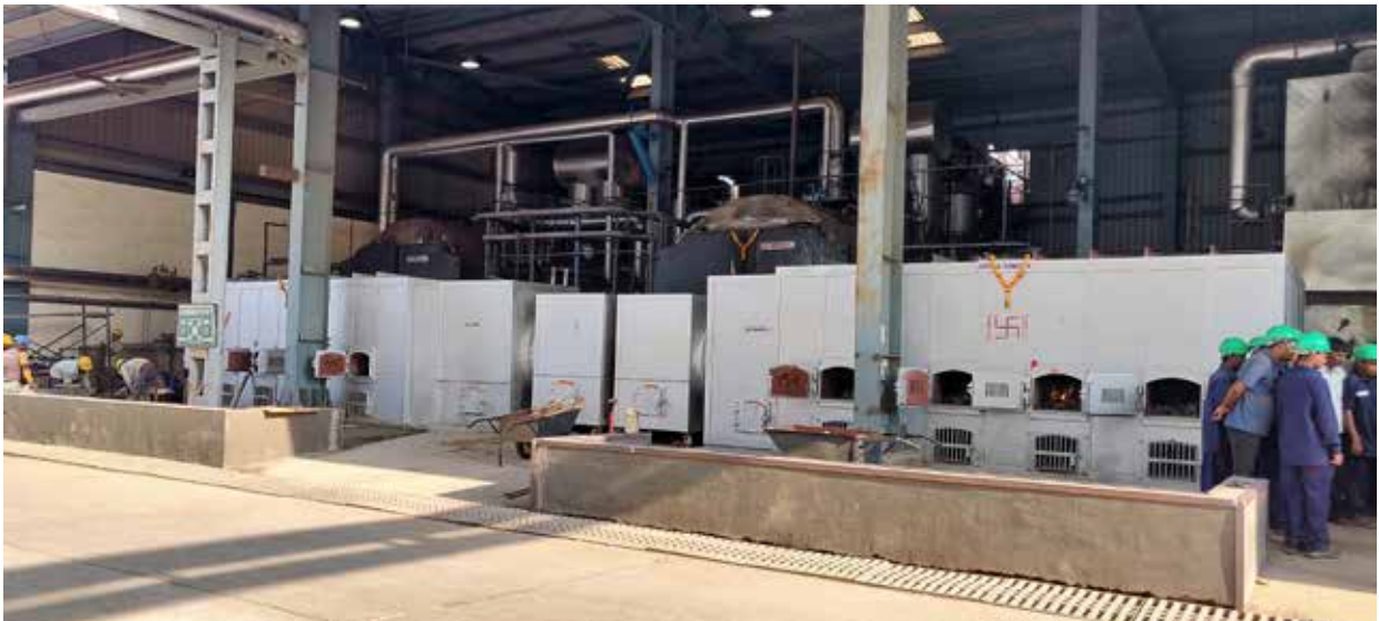
Briquette boiler at Ambernath factory
