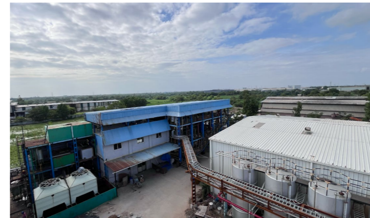
Kheda Plant - Gujarat
